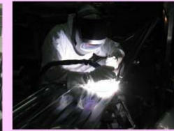
Pumping Port Welding
